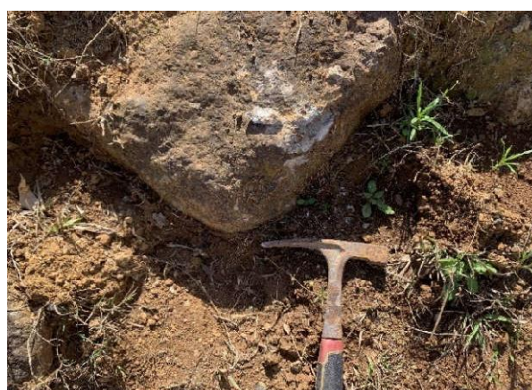
Outcropping basalt boulders were estimated to be of at least high strength.
